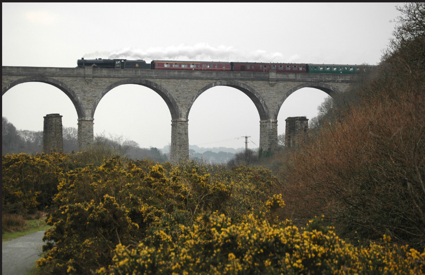
ABOVE: Just north of Perranwell on the Falmouth branch is the distinctive 253 yard long Carnon New Viaduct that spans the valley of the same name. The masonry pillars of a previous structure are well in evidence as No. 45407 heads for Truro from Falmouth Docks with 'The Falmouth Packet' on 25 March.
